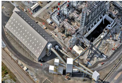
Refinery Services, BP Whiting
