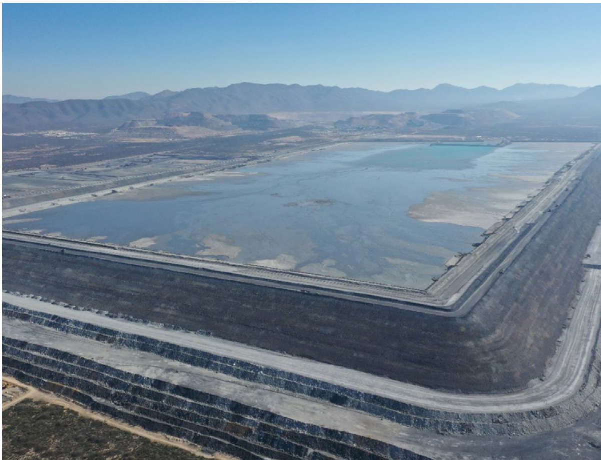
Photo: Presa de Jales, Peñasquito, Mexico
