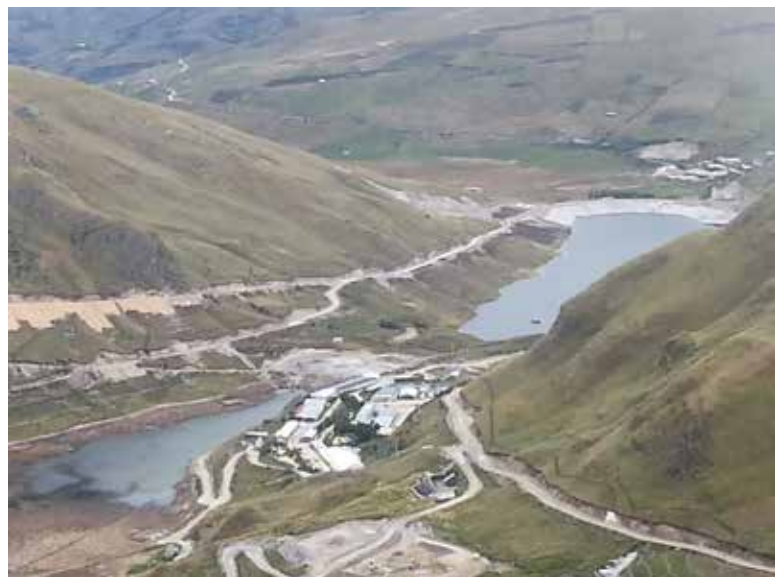
Reservoir is located in upper right and sediment control structure is in lower left.
