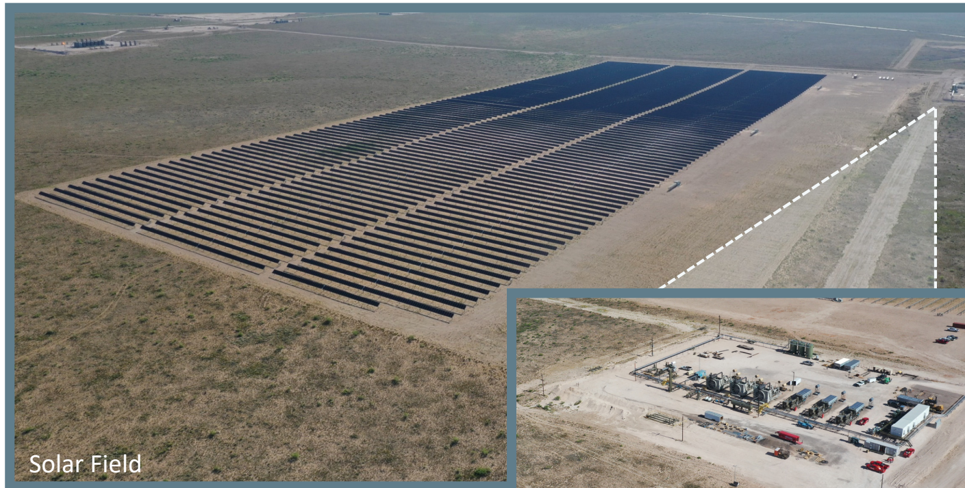
Solar/Natural Gas Hybrid Compression
