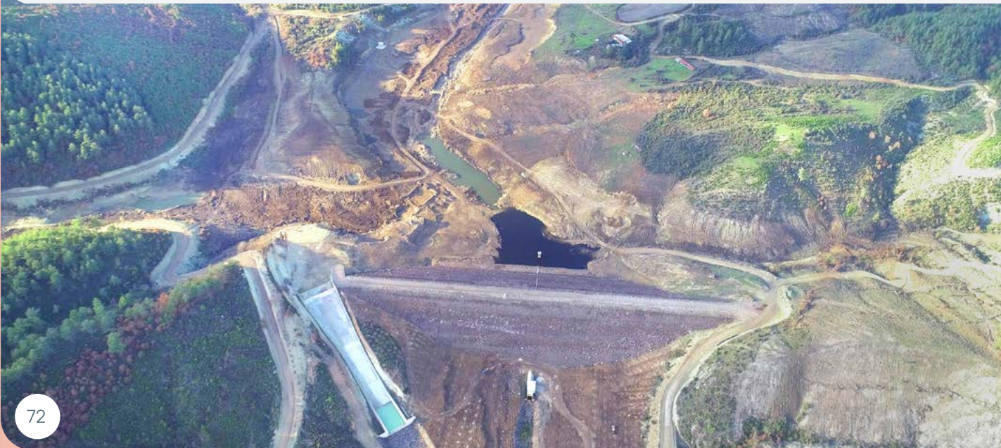
The Altınzeybek-2 water reservoir, built by Alamos near the Kirazlı project, Turkey.
