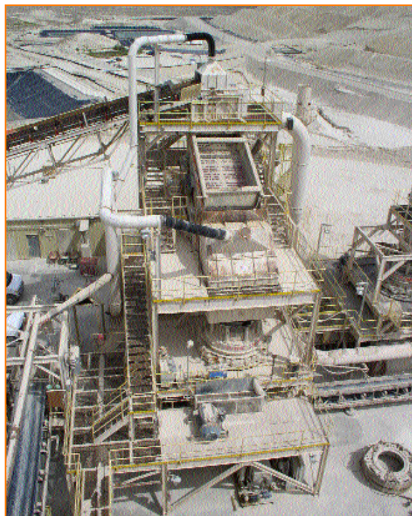
Transfer tower – 7' standard discharge to 7' shorthed – coarse ore stacker in upper left corner
