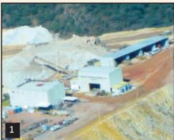
1 Upgraded Site Infrastructure
