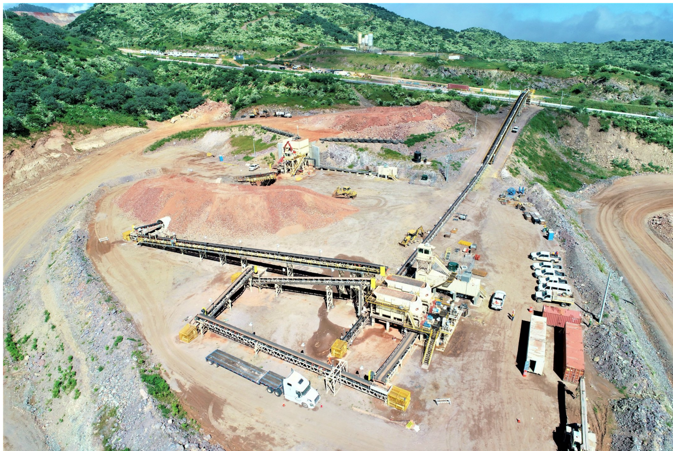
Cerro Pelon crushing circuit
